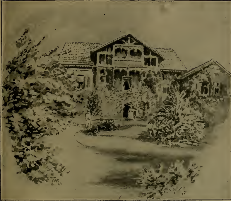
GREAT FRÖEN — THE DWELLING-HOUSE
