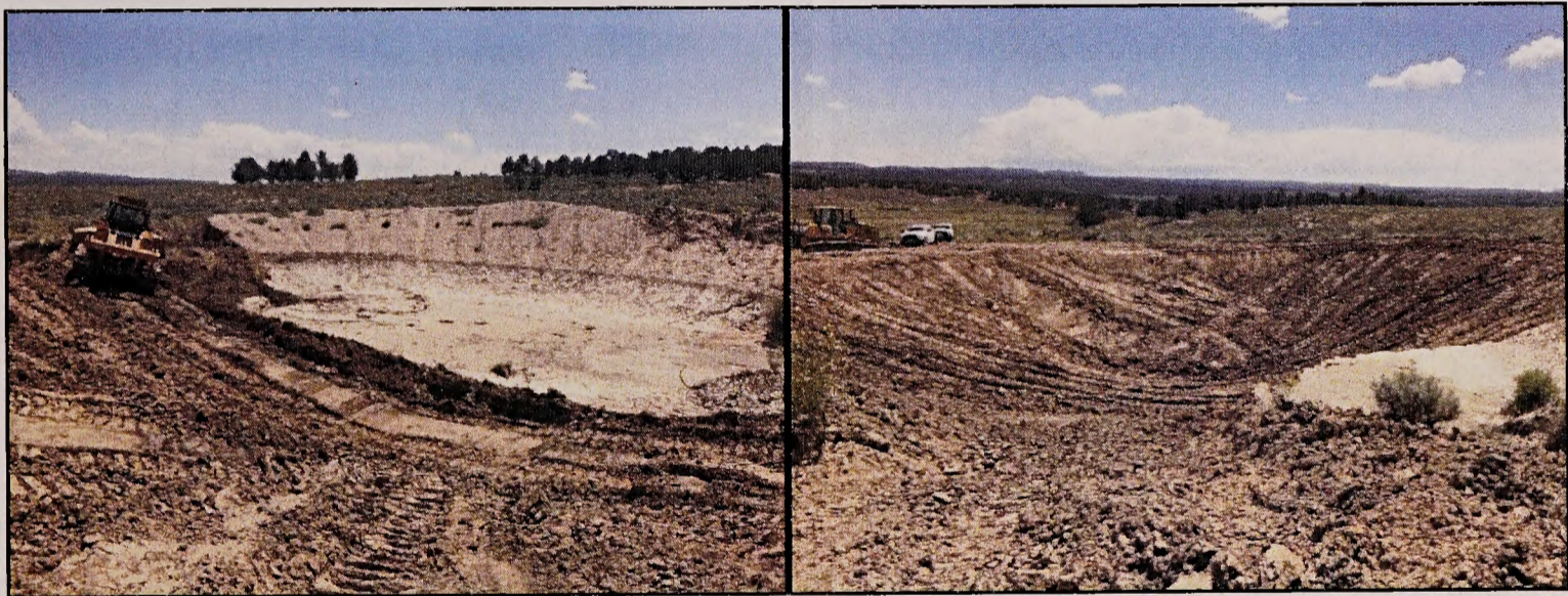
Figure 20 - Thompson Draw before (left) and after (right) maintenance.
