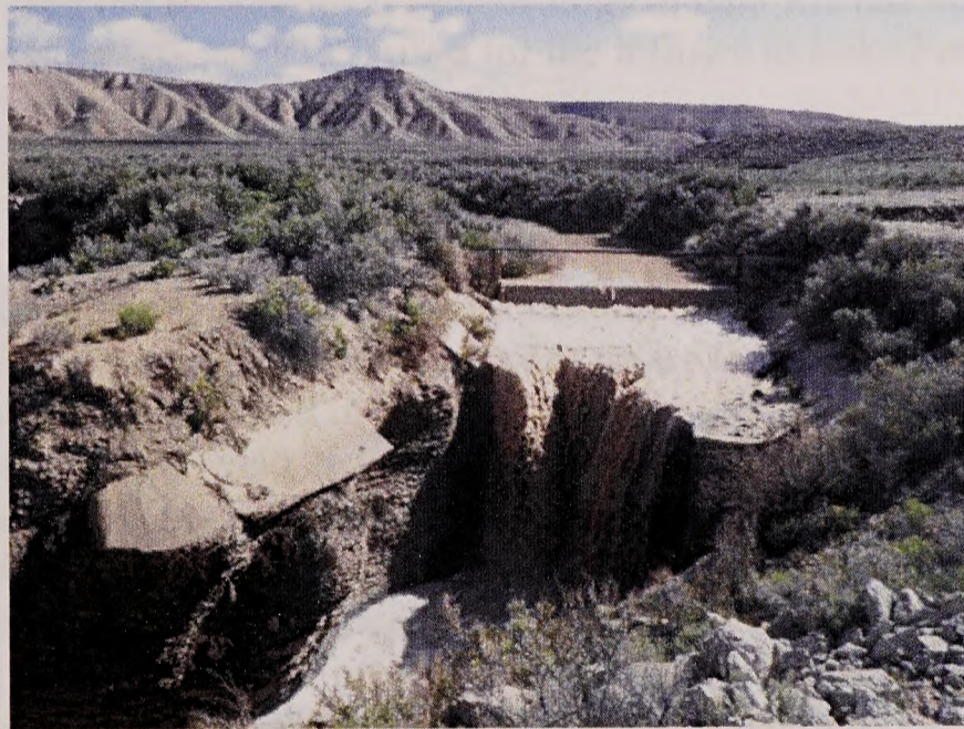
Figure 26 - The Pierotto Drop structure
