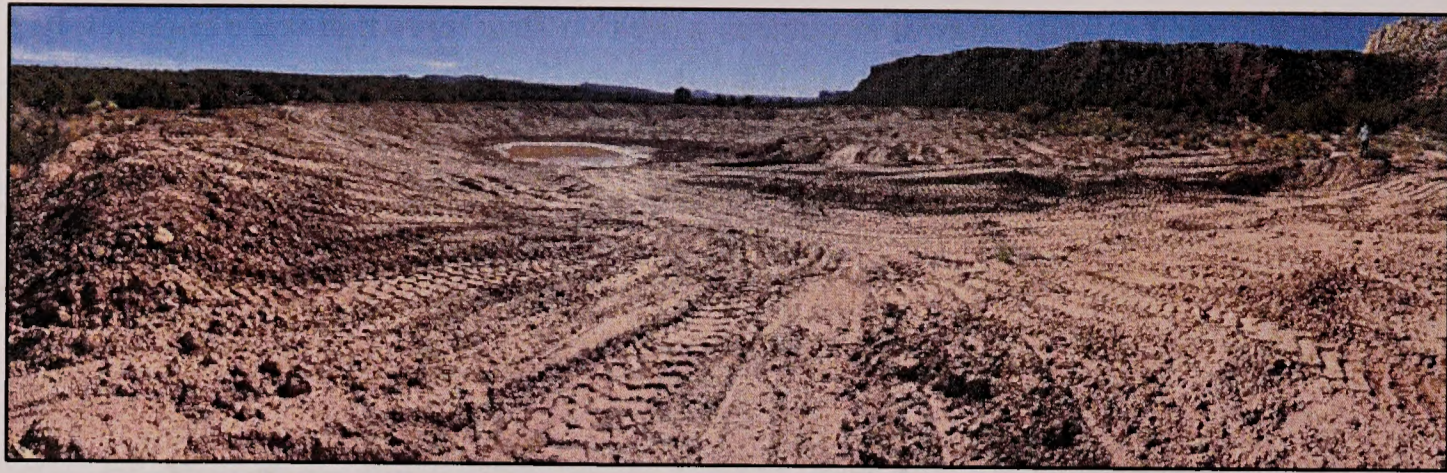
Figure 24 - Large salinity control structure near the Wolverine Loop Road in the Circle Cliffs. This structure was cleaned in August 2017. The structure captures saline sediments from Chinle Formation outcrops to the west.
