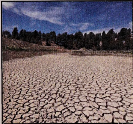
Figure 19 - Dry Wash Structure FY2018
