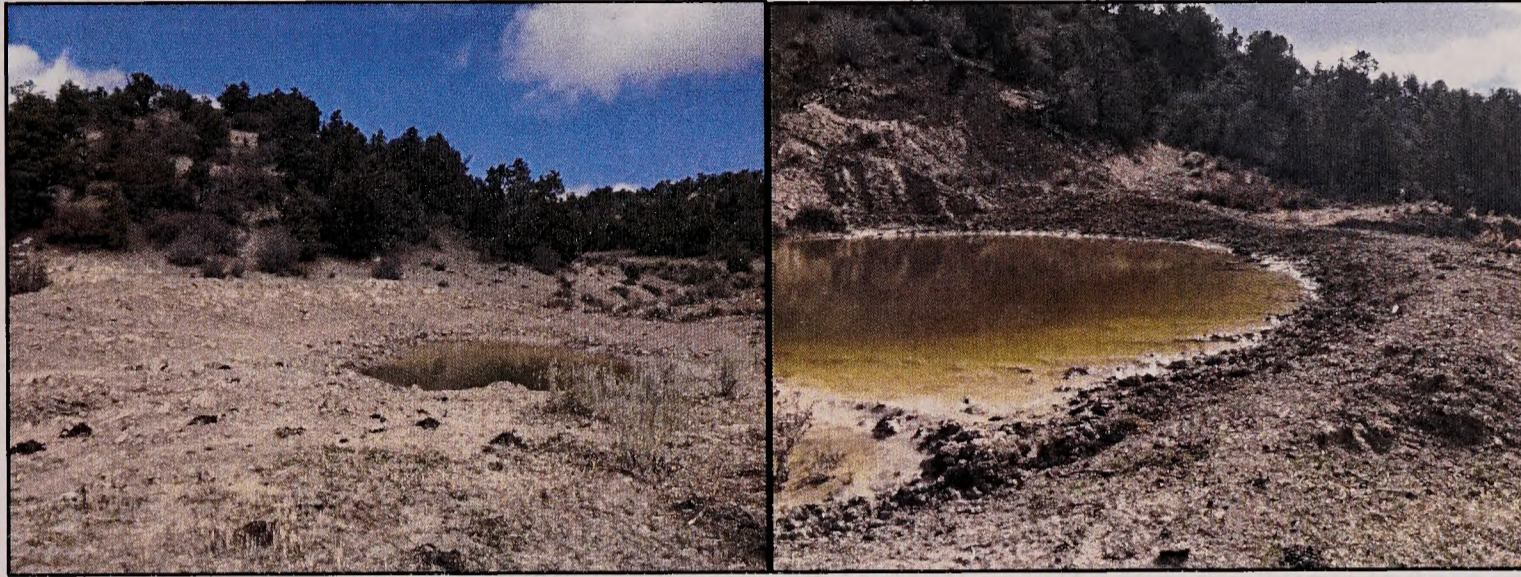
Figure 23 - Upper Sink Valley structures 1 (left) & 2 (right) after catching water and sediment.
