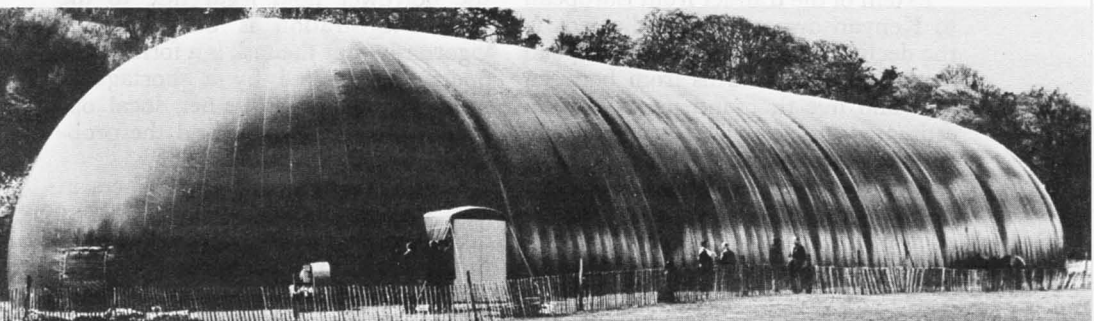
Inflatable plastic warehouse built for Maize Marketing Board in Kenya. Warehouse holds 5,000 tons of bagged maize (corn). It is portable, moisture proof, and can be fumigated.
