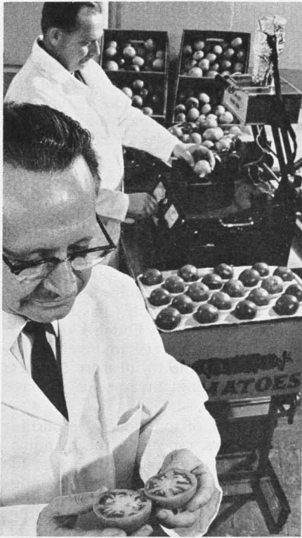
Left, Multiple Wavelength Difference Meter tells how ripe a tomato is without cutting it. Below, colorimeter developed by USDA measures quality of tomatoes for juice more accurately than can be done by eye.
