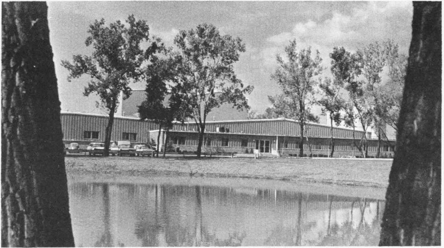
Pond designed to prevent water damage and beautify factory site in Ontario County, N.Y.
