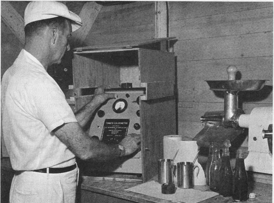
Left, Multiple Wavelength Difference Meter tells how ripe a tomato is without cutting it. Below, colorimeter developed by USDA measures quality of tomatoes for juice more accurately than can be done by eye.
