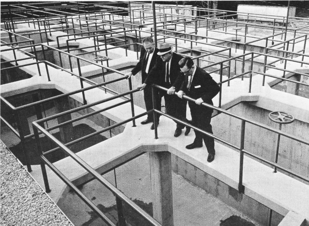
Filtration tanks of new water system in Denton, N.C.
