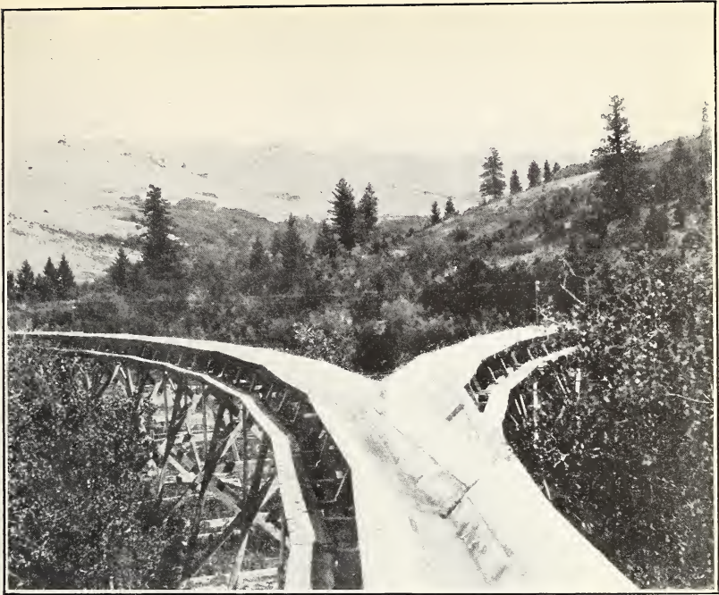
FIG. 1.—A BRANCH FLUME, SHOWING METHOD OF CONNECTION WITH MAIN FLUME. In this case the branch is closed off by the use of two "lining" blanks.
