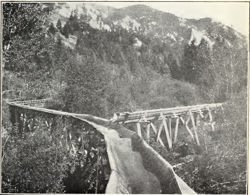
FIG. 2.—A FEEDER FROM A SIDE CREEK. Notice cheap form of construction.
