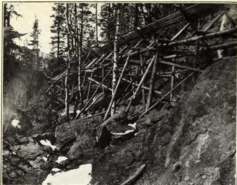
FIG. 1.—A FLUME IN THE CONSTRUCTION OF WHICH SMALL ROUND TIMBER WAS USED FOR EVERYTHING EXCEPT THE "BOX."
