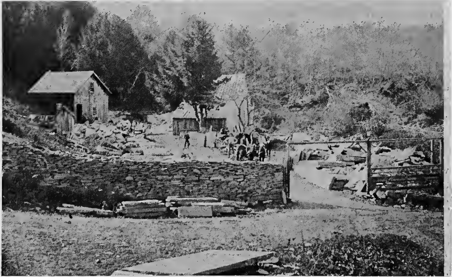
THE APPROACH TO JOHN E. MILLER'S QUARRY.
