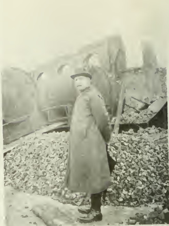
Fig. 5. Wrecked boilers and boiler house.
