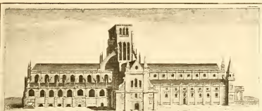
North-west view of Old St Paul's Church after the Spire was destroyed by Lightning.
