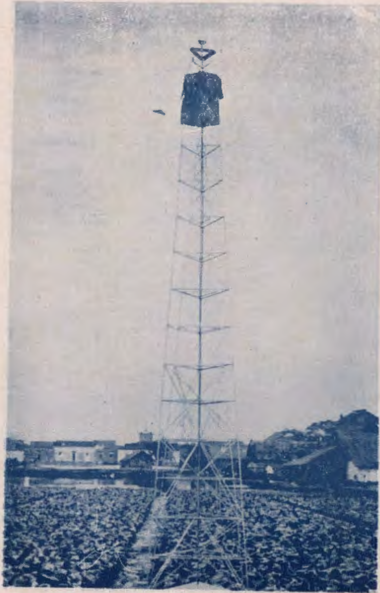
New Triangulation Steel Tower, 113ft
