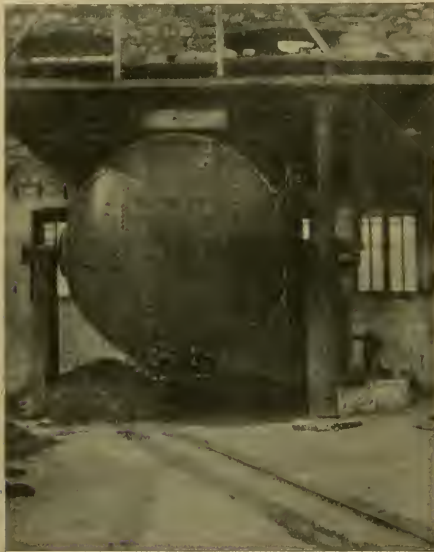
Fig. 4.—Peat digester, peat paper factory, Celbridge, co. Kildare.
