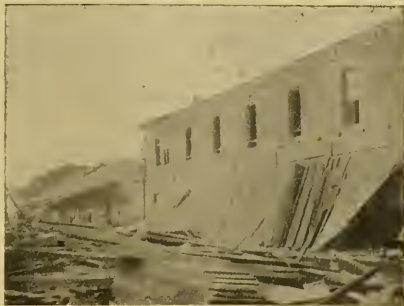
FIG. 1.—Railway station wall facing south.
