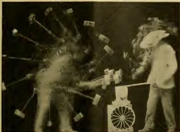
FIG. 1.—Composite photograph of a smith and striker for one swing of the hammer.
