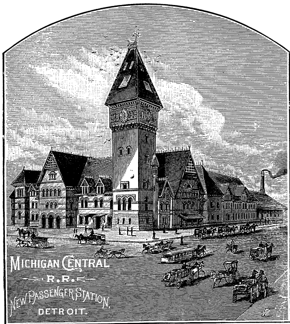
MICHIGAN CENTRAL DEPOT.
