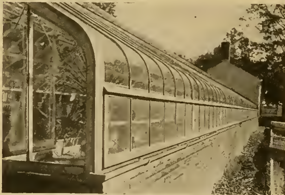
At the base of the curved eave, is an angle iron, to which the side sash are hinged.
