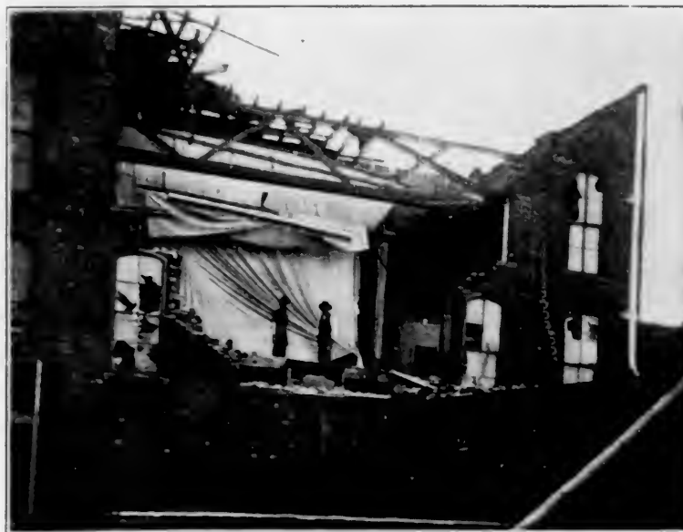
Above is a representation of the wrecked Madison Opera House at Tuscola, Ill., caused by a severe wind and rain storm that passed over the city on May 30. It shows the rear of the theatre. The picture was taken by Manager H. S. Bassett's son, J. F., for The Billboard.
