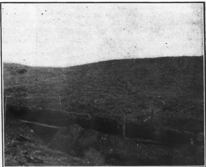
FIG. 6. CLOSE VIEW OF FIG. 5. POST IN CENTER OF PICTURE IS VERTICAL
