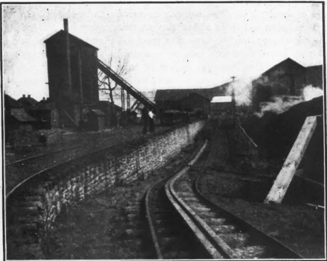
FIG. 2. RACK-RAIL ON EMPTY CAR TRACK. SHORT GRADE OF 14 PER CENT., SWITCH AT BOTTOM
