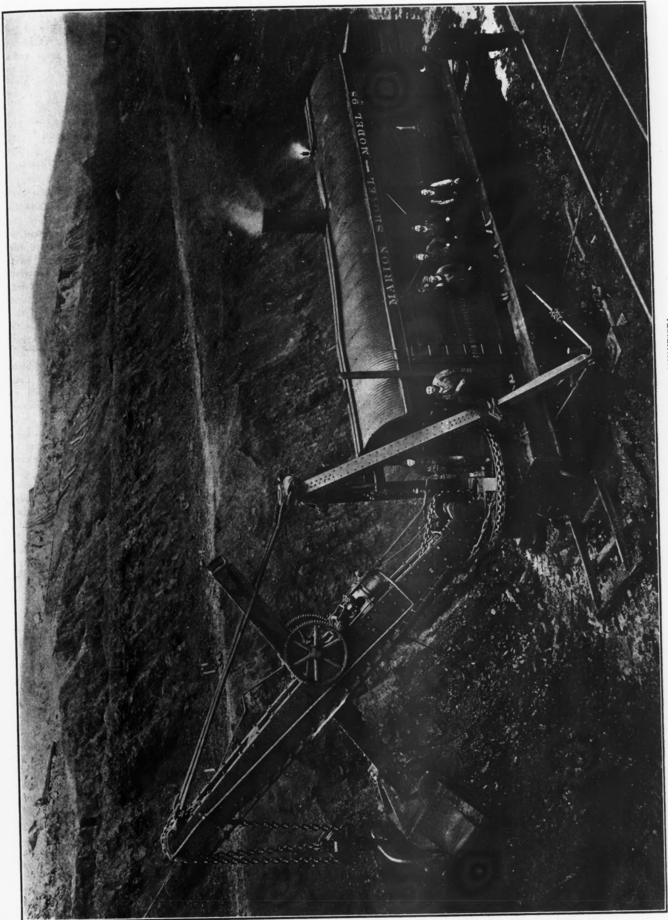
STEAM SHOVEL AT WORK AT STEVENSON MINE, MINNESOTA
