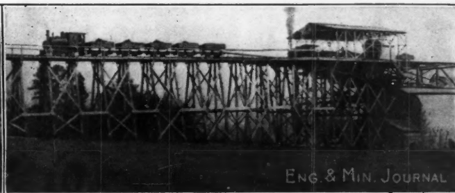
NEW SLOSS-SHEFFIELD PLANT
