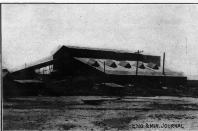
GENERAL VIEW OF DOME MILL
