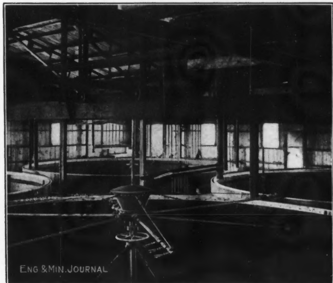
LEACHING TANKS AT DOME MILL
