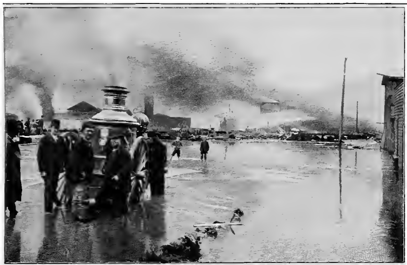
From foot of Monroe Street, looking South, at 11 A.M., Sunday, June 5, 1892
