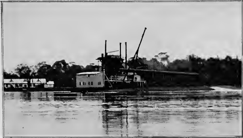
Machine Shop and Railroad Camp Number 1, showing one of the Dredges at Work on the Nicaragua Canal
