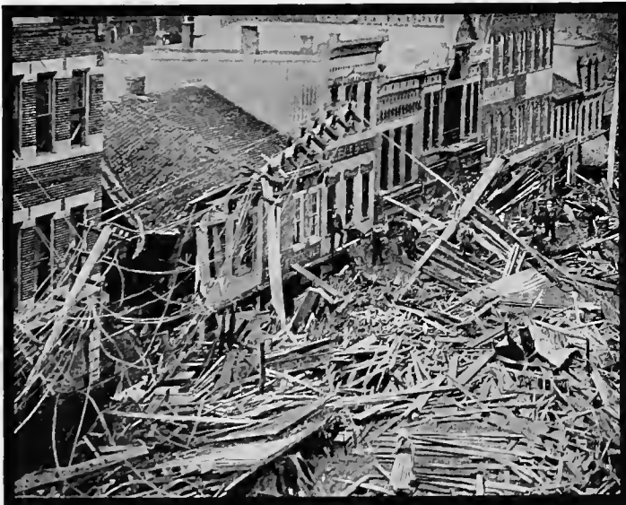
MAIN STREET, JOHNSTOWN, AFTER THE FLOOD
