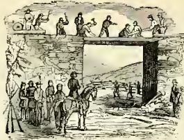
TRUEN'S REPAIRING THE MILLENTON BRIDGE, ON THE RAILROAD FROM ANAPOLIS TO WASHINGTON.
