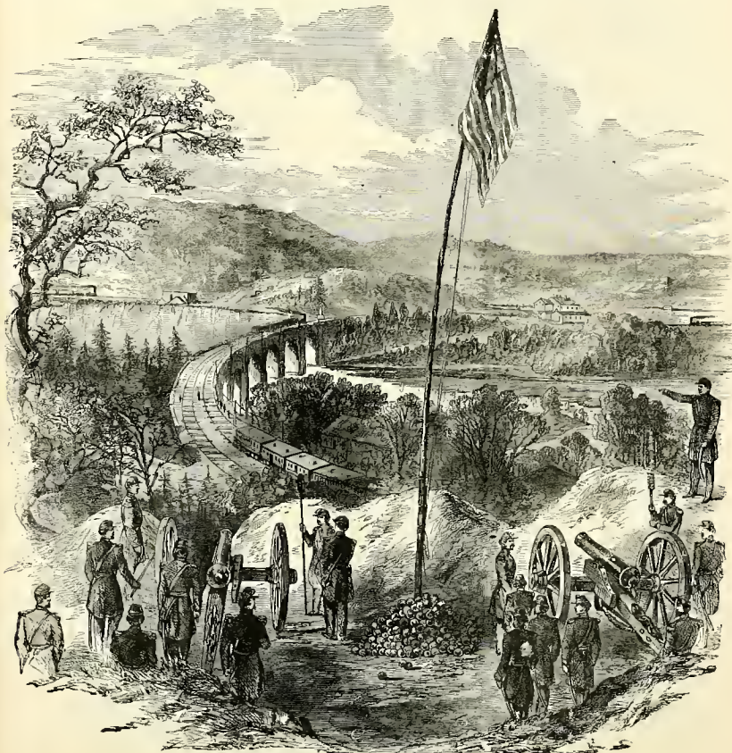
THE BOUQUET BATTERY, COMMANDING THE VIADUCT OVER THE PATAPSCO RIVER, ON THE BALTIMORE AND OHIO RAILROAD, NEAR THE RELAY HOUSE.
