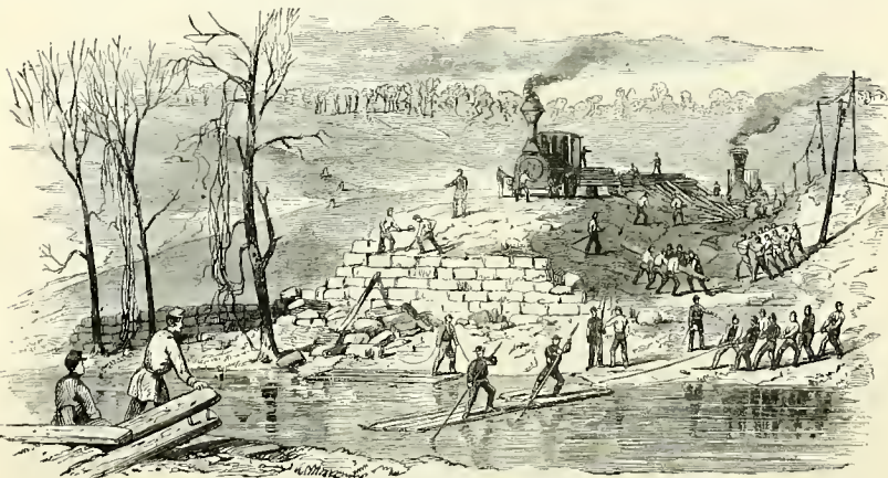
THE FEDERAL SOLDIERS REPAIRING THE RAILROAD BRIDGE OVER GOOSE CREEK, DESTROYED BY THE CONFEDERATES IN THEIR RETREAT.
