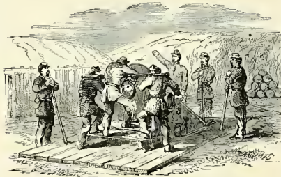
MORTAR PRACTICE—PUTTING IN THE SHELL.
