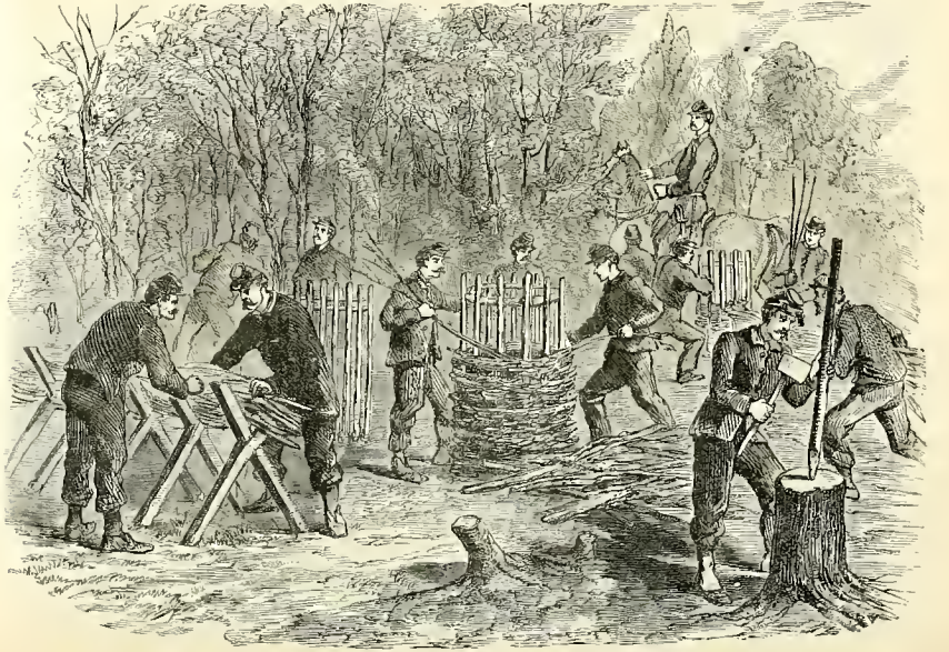
CAPTAIN MULLEN'S BATTERY, SEVENTY-SEVENTH PENNSYLVANIA REGIMENT, MAKING FASCINES AND GABIONS FOR BREASTWORK.
