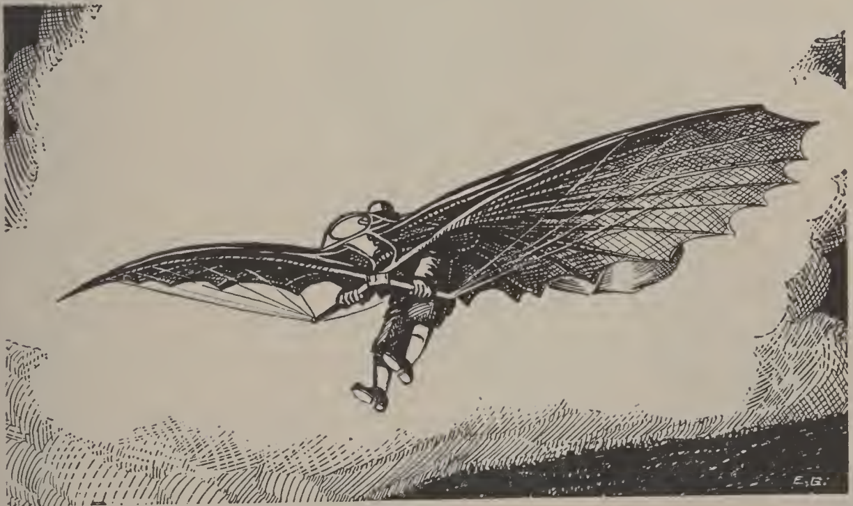
THE LILIENTHAL BROTHERS HAD MADE GLIDERS, LIKE THIS ONE, WHICH HAD NO ENGINES.
