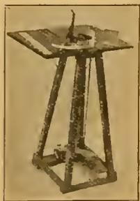
The best Machine on earth for Fastening in Starters and Pressing the Sections together; it rapidly moves the Foundation In, cuts it of the desired length and presses it on—all at one operation. With one of these Machines one man can do more work in a first-class manner than four men with any of the other machines now made. If you want one this season, order at once.
