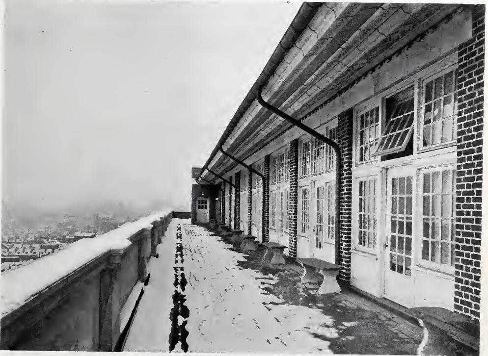
Terrace Outside Recreation Room.
