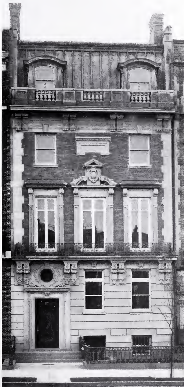
THE C. N. WALLACE HOUSE, Boston, Mass. Kilham & Hopkins, Architects.
