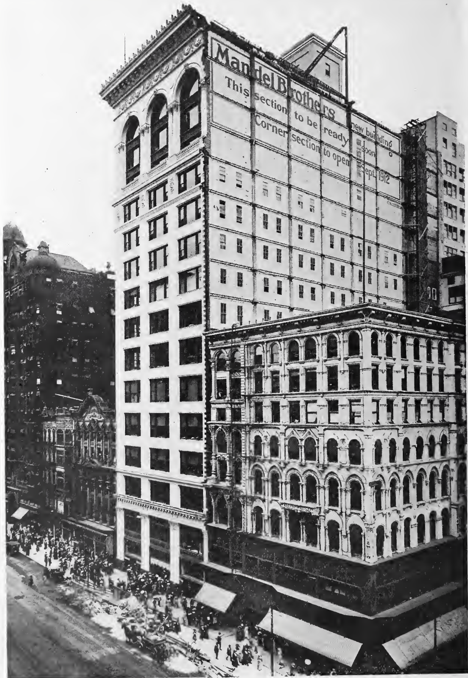
FIRST SECTION MANDEL BROS. BUILDING, N. E. COR. STATE & MADISON STS., CHICAGO, ILL. HOLABIRD & ROCHE, ARCHITECTS.
