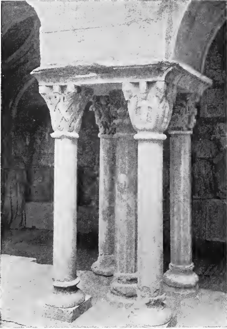
CLUSTER OF COLUMNS AT A CORNER IN GERONA CLOISTERS.
