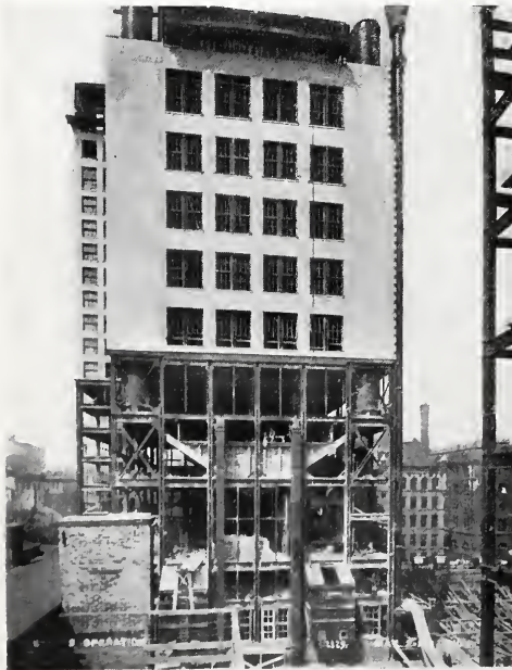
POWER BUILDING FROM COURT, SHOWING COAL-BUNKER FIRING COAL CONVEYORS, SMOKE-STACKS, ASH BINS, BRICK FACING ON COURT SIDE, ETC.
