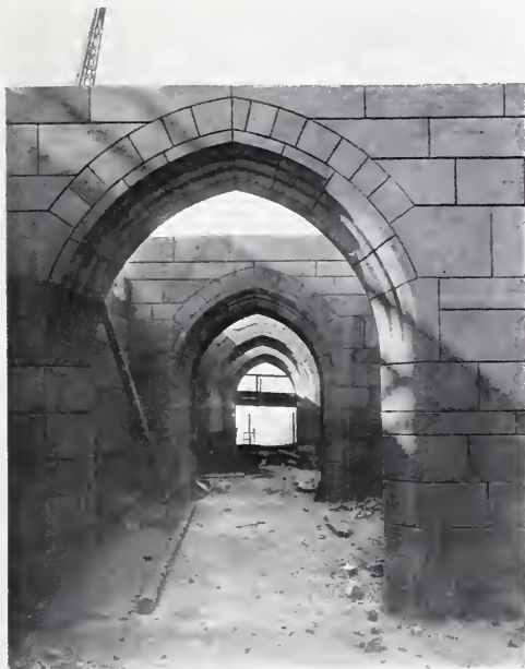
SOUTH TRIFORIUM LOOKING WEST.
