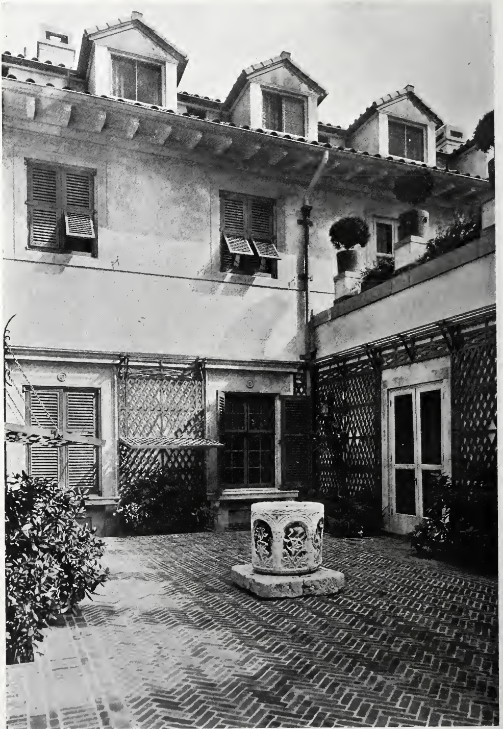
THE SOUTH COURT—HOUSE OF HAROLD F. McCORMICK, ESQ., LAKE FOREST, ILL. CHARLES A. PLATT, ARCHITECT
