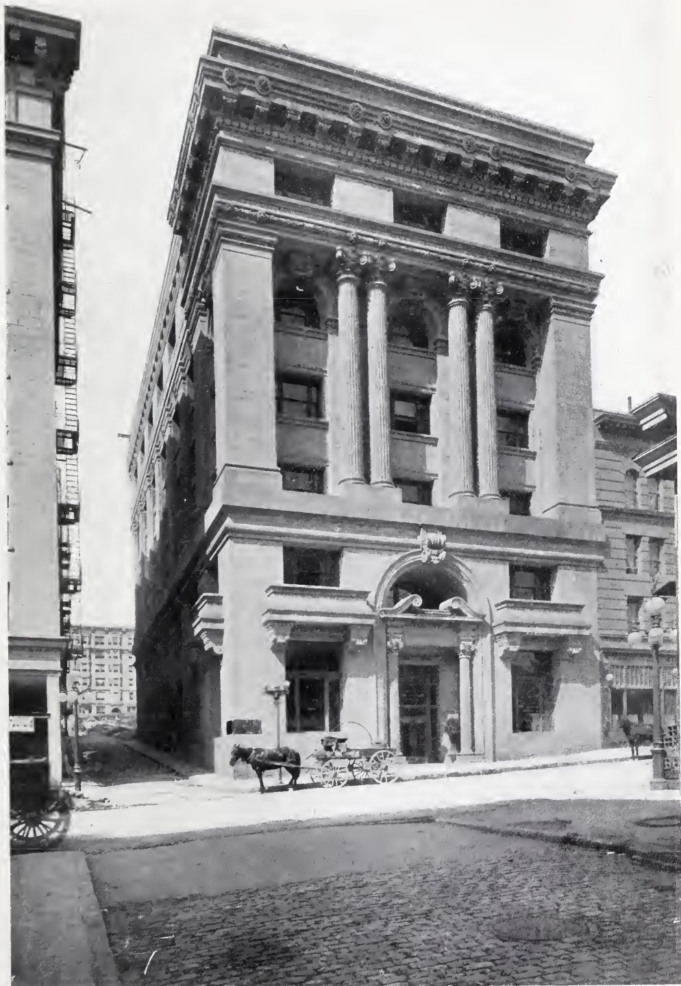
THE HOME TELEPHONE COMPANY BUILDING, SAN FRANCISCO, CALIFORNIA. COXHEAD & COXHEAD, ARCHITECTS.
