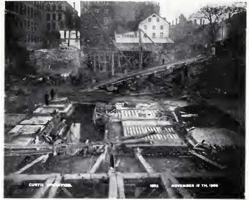
COFFERDAM AND FOUNDATION GRILLAGES.
