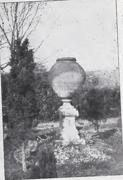
FIGS. 16, 17, 18 AND 19—CONCRETE USED FOR GARDEN ORNAMENT.
