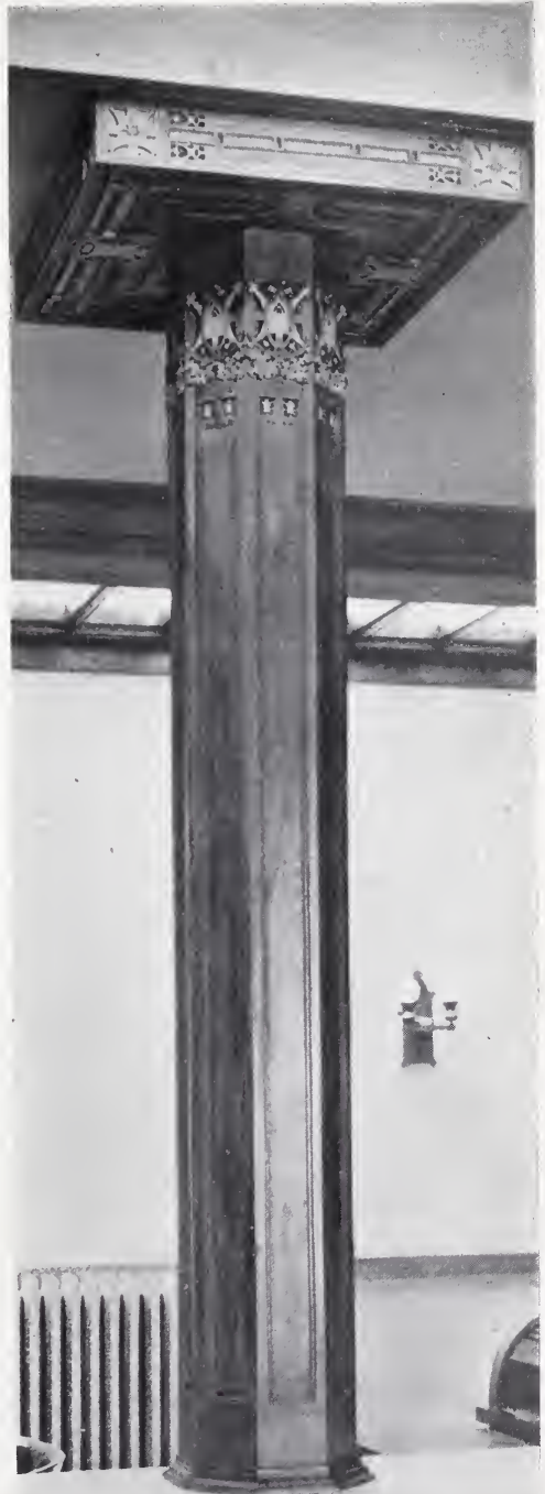
DETAIL OF COLUMN IN BANKING ROOM—THE PEOPLE'S SAVINGS BANK. Louis H. Sullivan, Architect.
