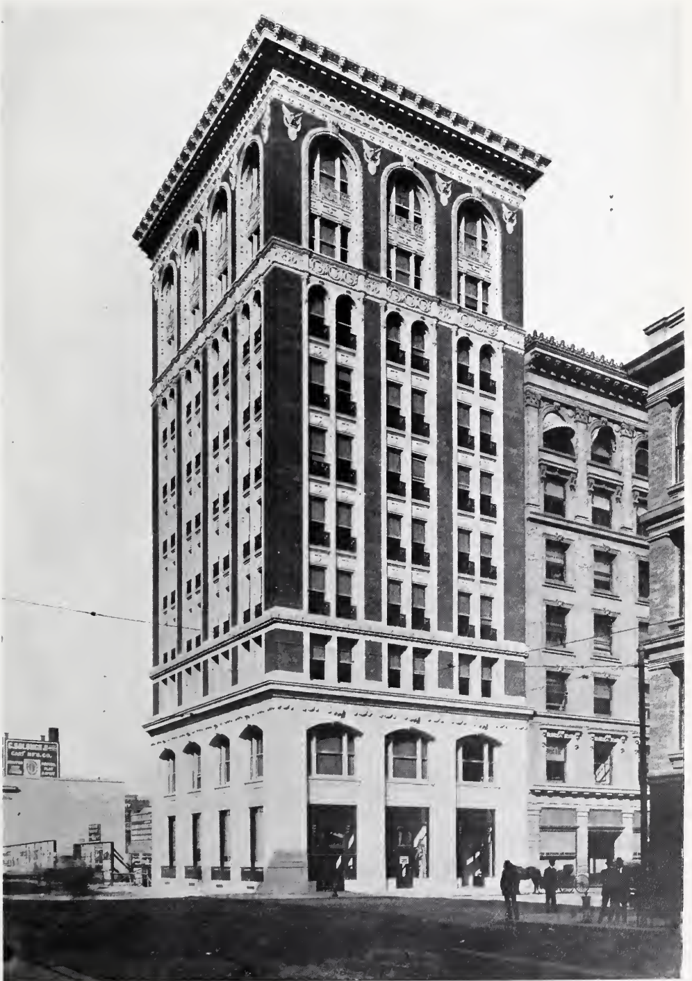
THE NEWHALL BUILDING, SAN FRANCISCO, CALIFORNIA. LEWIS HOBART, ARCHITECT.
