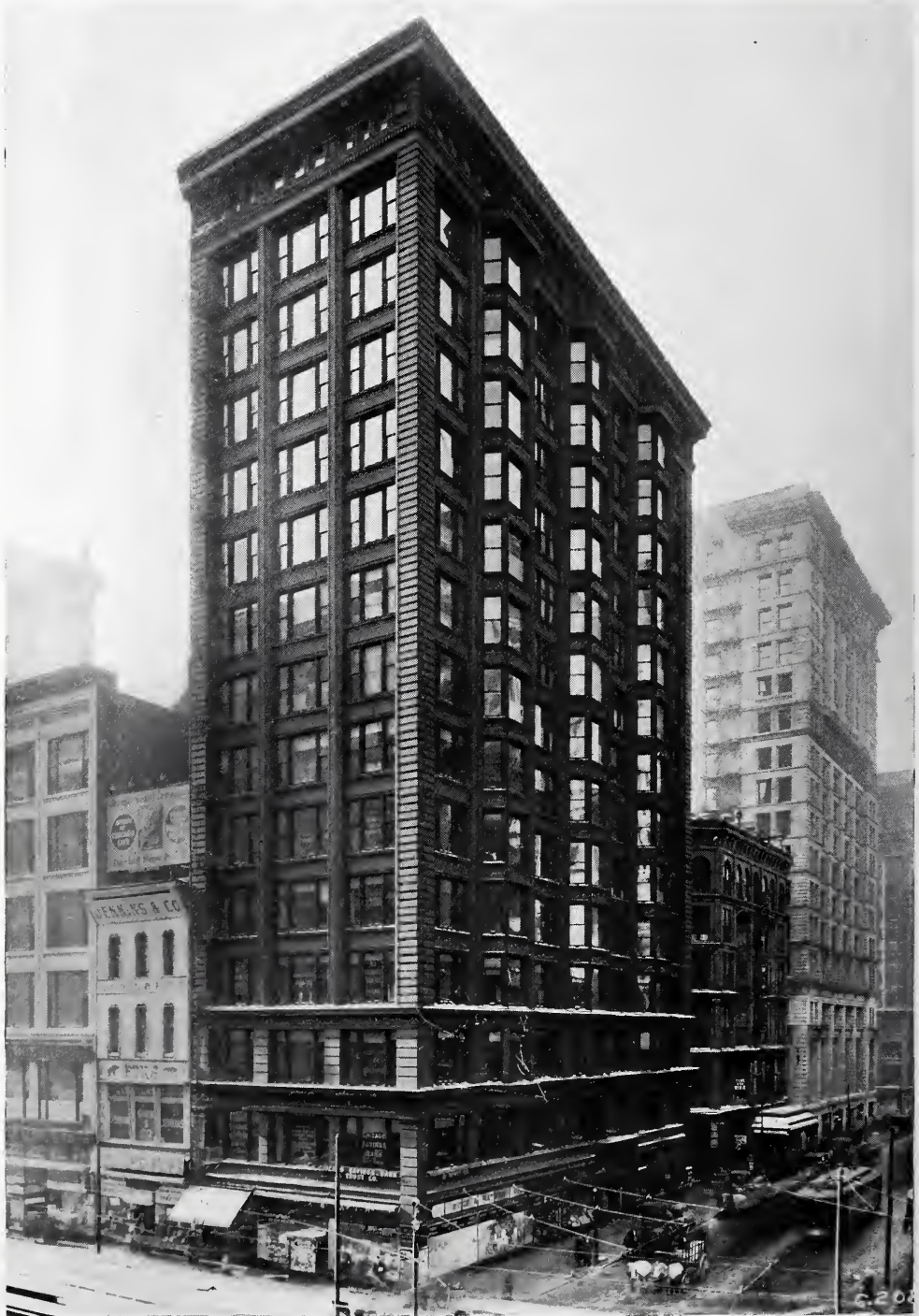
CHICAGO SAVINGS BANK BUILDING. HOLABIRD & ROCHE, ARCHITECTS.
