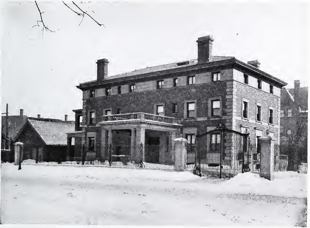
RESIDENCE FOR MR. MILVILLE N. ROTHSCHILD, 37TH ST. AND MICHIGAN AVE., CHICAGO.
