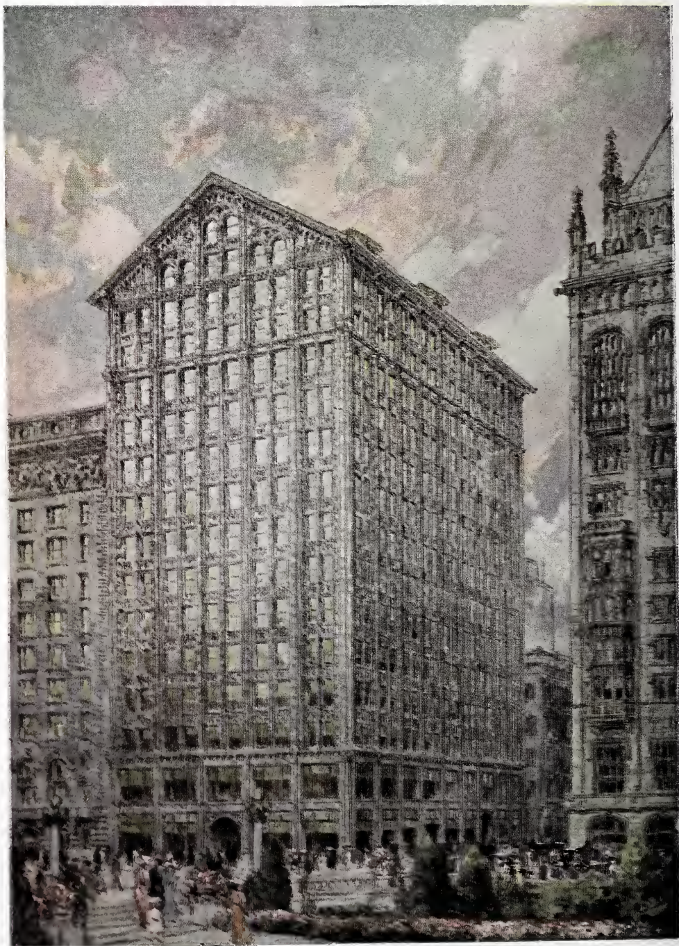
THE MONROE BUILDING, MICHIGAN AVE., CHICAGO, ILLINOIS. HOLABIRD & ROCHE, ARCHITECTS.
