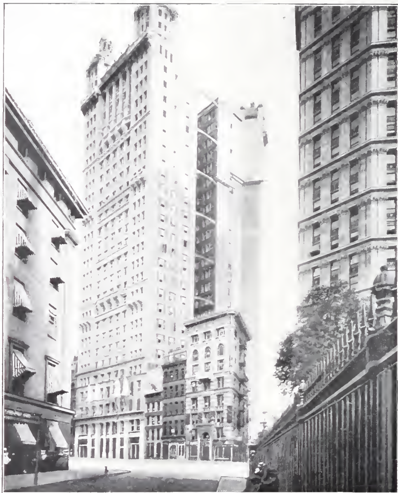
THE PARK ROW BUILDING.
