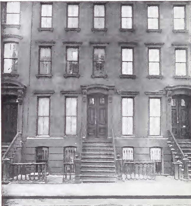
NO. 238 EAST 51ST STREET.
