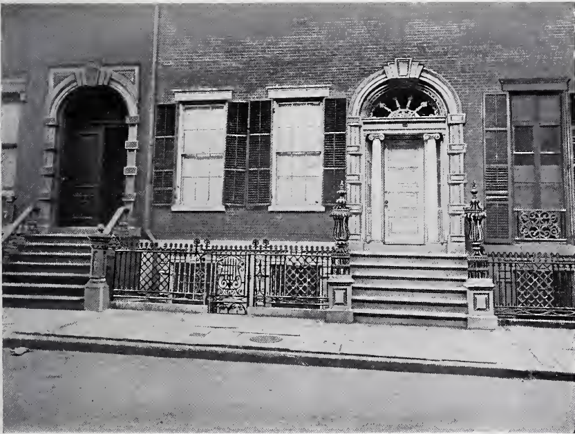
NOS. 27 AND 29 EAST 4TH STREET.
