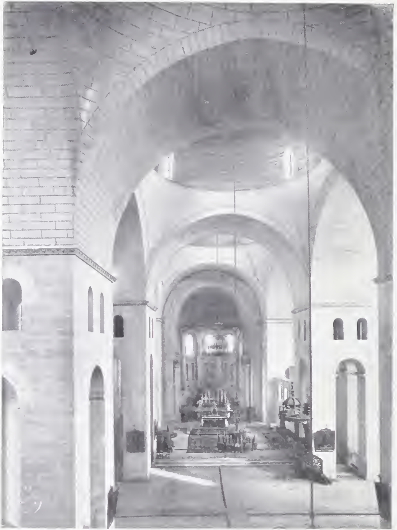
S. FRONT, PERIGUEUX. (View of Interior, from the West.)
