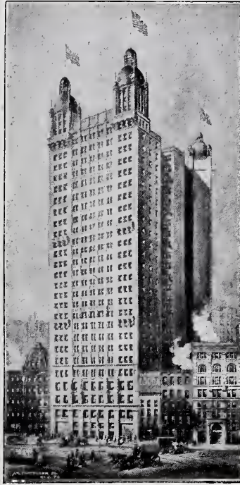
THE PARK ROW BUILDING.
