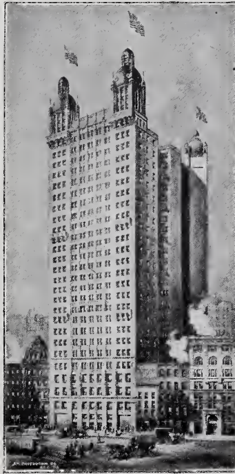
THE PARK ROW BUILDING.
