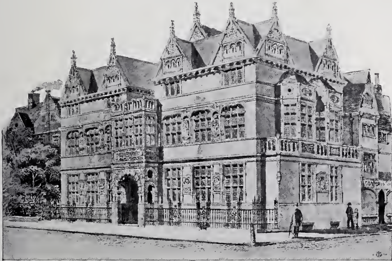
272. This design is rescued from the charge of "double composition" by the prominence of the projecting porch.
