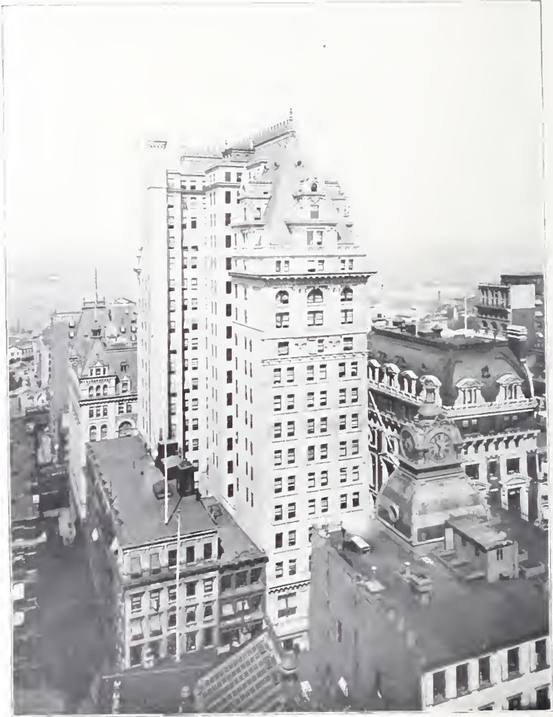
THE WASHINGTON LIFE BUILDING. (From the East.)
