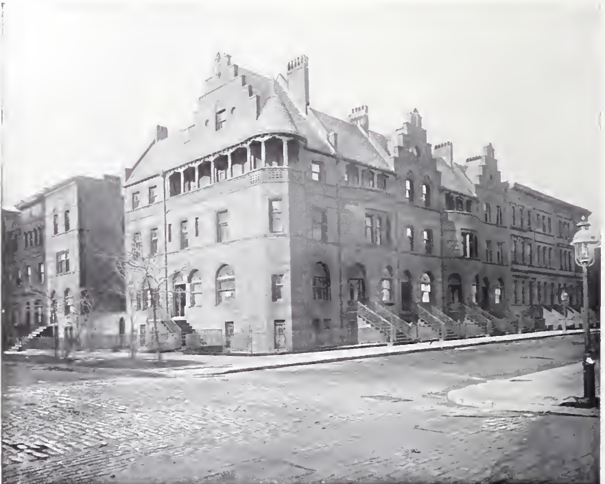
SOUTHWEST CORNER OF WEST END AVENUE AND 83D STREET.
