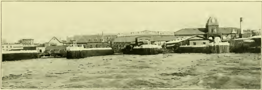
LONG ISLAND RAILROAD FERRIES AND SLIPS.
