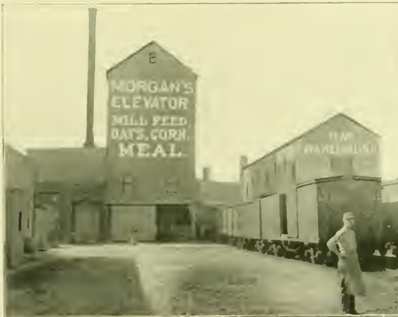
VIEW OF THOMAS MORGAN'S ELEVATOR AND YARDS.
