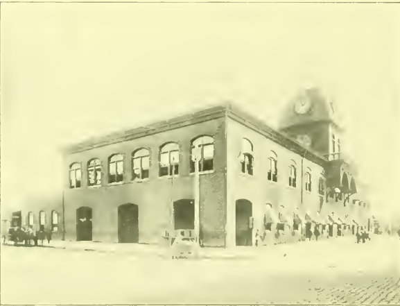
LONG ISLAND RAILROAD STATION.
