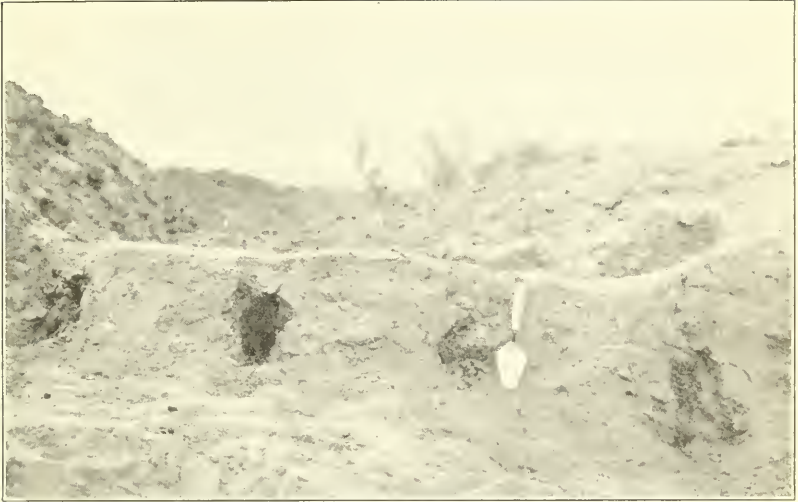
a , Charred posts in adobe wall, illustrating method of construction
