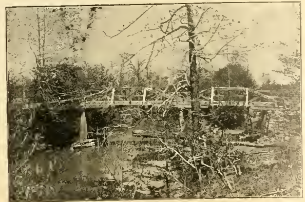
Reed's Bridge, National Military Park.
