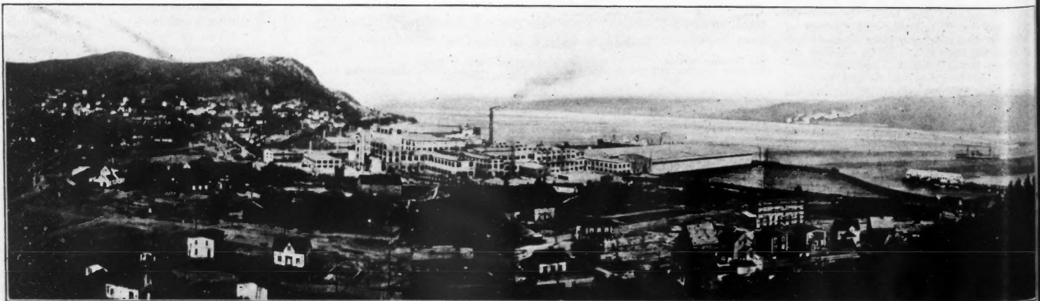
Panorama Snapshot of New Plant of the Newfoundland Power and Paper Co., Corner Brook, Newfoundland
