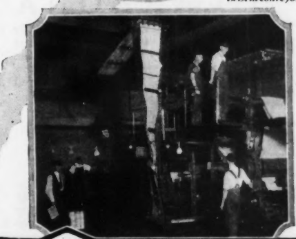
Knoxville-Sentinel Press Room, showing twist in conveyor
