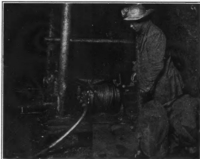
"TURBINAIR" HOIST USED IN SLUSHING
