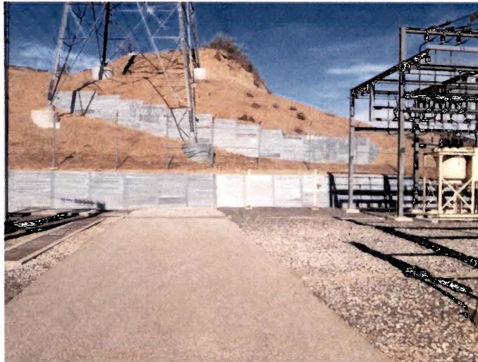
Typical soldier pile wall.
