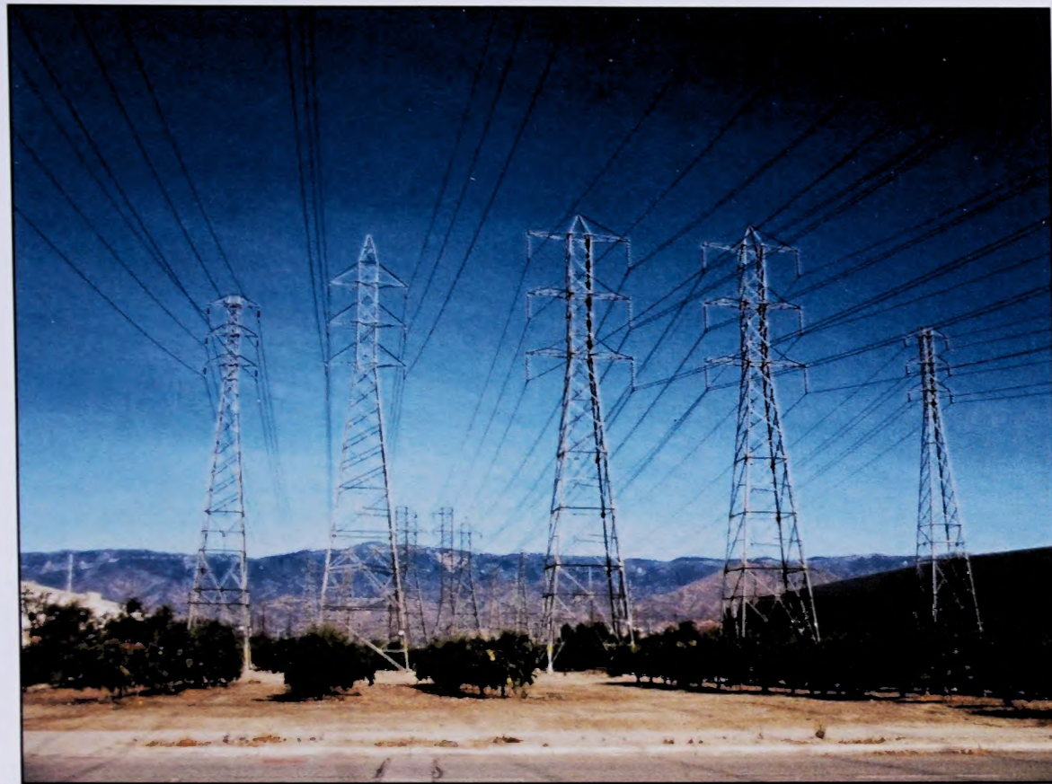
Photo 1. Segment 1 looking south from San Bernardino Substation
