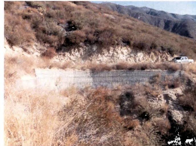
Typical welded wire wall.
