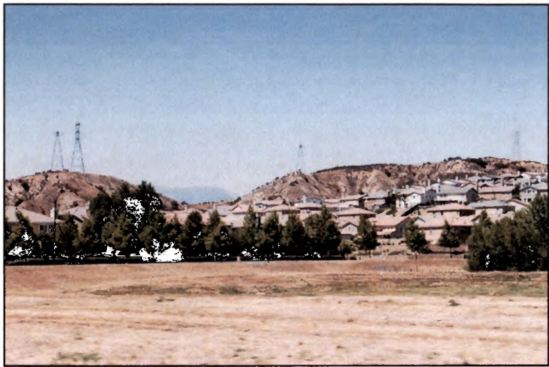
Photo 7. Segment 3 west of El Casco Substation from San Timoteo Canyon Road
