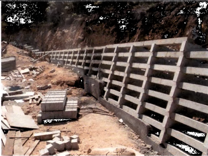
Typical concrete crib wall.
