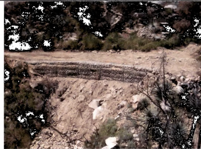
Typical gabion wall.
