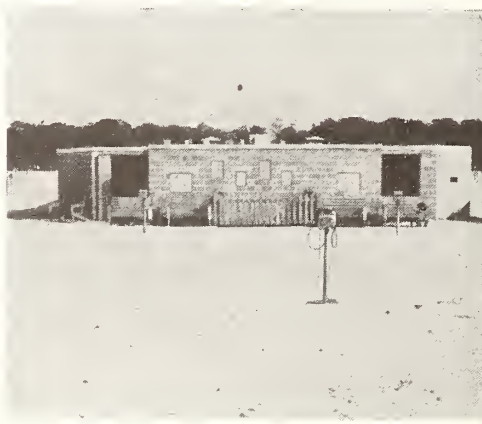
Screen-side view of the projection-toilet-concession building of the Springfield drive-in. It is built of cement block.
