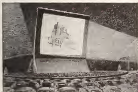
This new concave screen tower, designed for faithful and more brilliant picture reproduction, has been developed for prefabrication and national distribution. It is a current example of continuing engineering study by Park-In Theatres, Inc.
