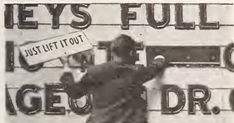
Ordinary lamps anywhere in the sign, easily accessible through "Remova-Panel".
