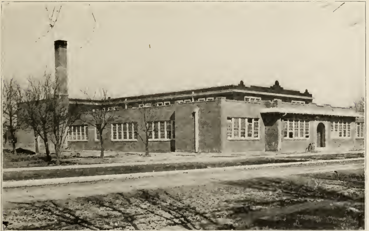
NEW HIGH SCHOOL BUILDING, PRYOR
