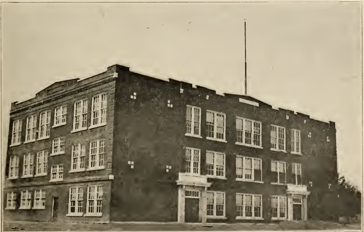
HIGH SCHOOL, NOWATA
