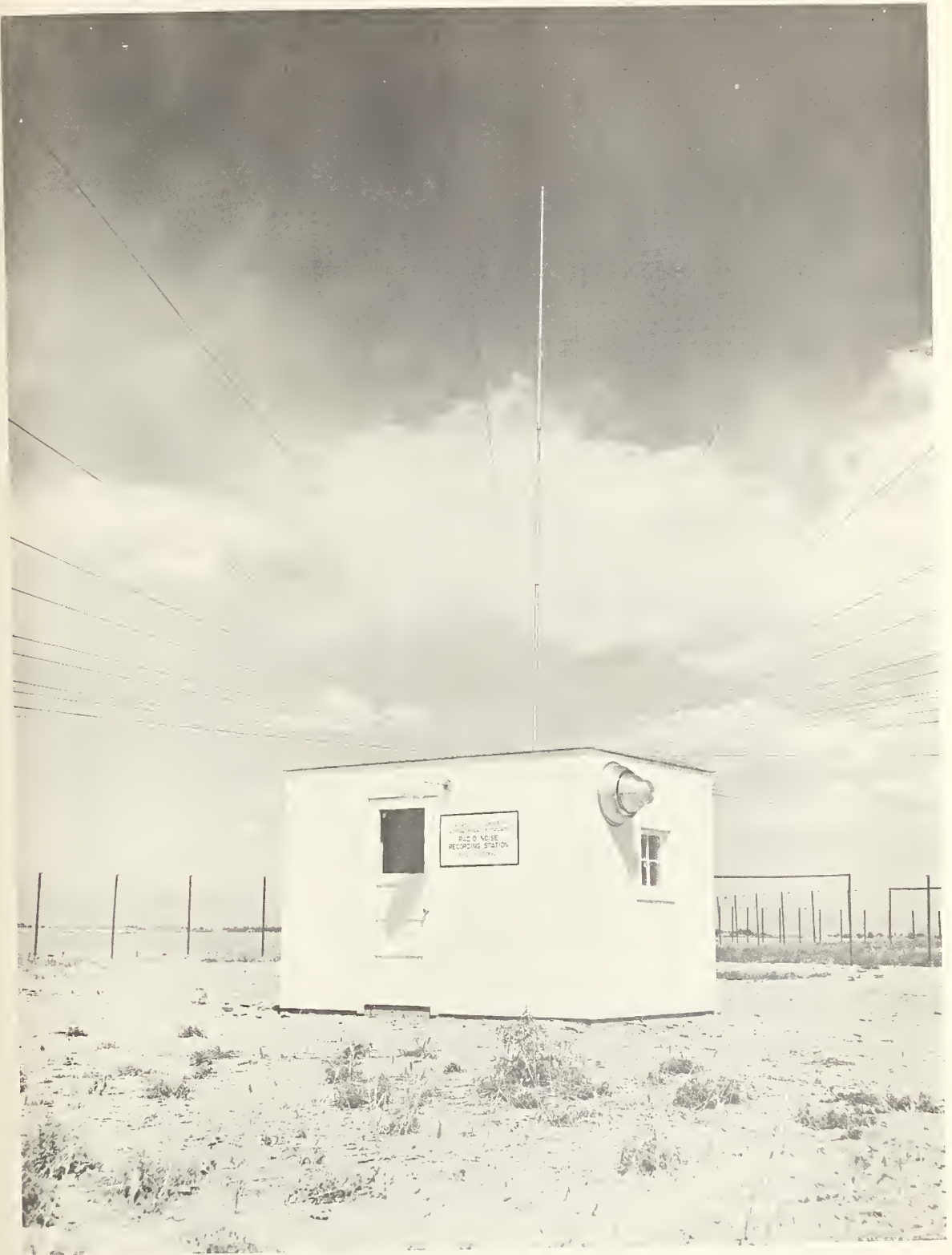
Radio Noise Recording Station
