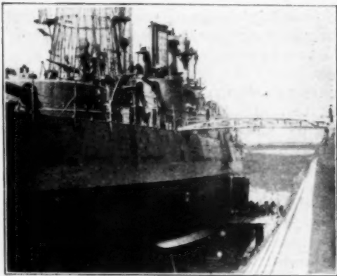
View Showing Position on Ship's Side
