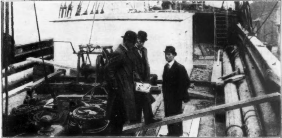
View of the Deck
