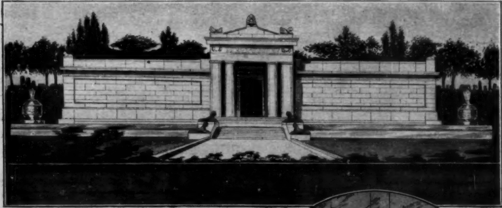
Mausoleum Under Erection at Cleveland
