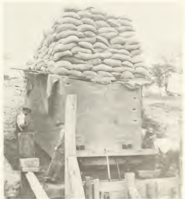
FIGURE 26—Concrete casing for lysimeter, weighted to 100,000 pounds, in partly excavated trench.
