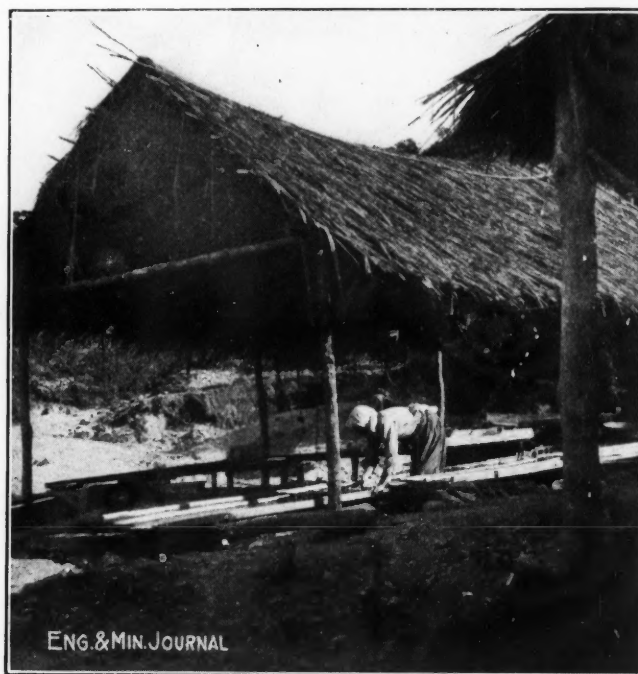
CLEANING SLUICES AFTER A MILL RUN
