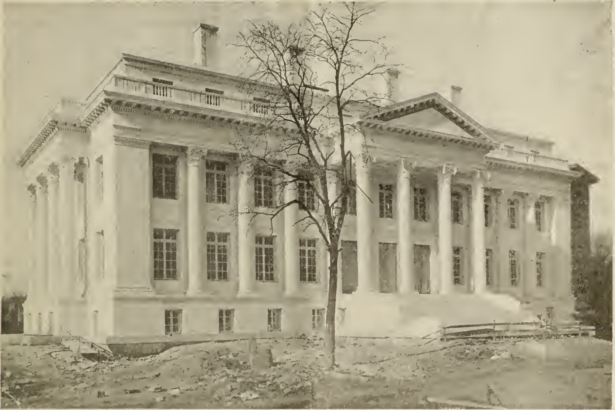
THE NEW RED CROSS BUILDING AT WASHINGTON, OCCUPIED BEFORE IT WAS COMPLETED
