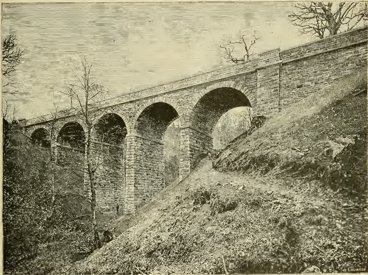
LOB GHYLL VIADUCT, YORKSHIRE, ENGLAND.
