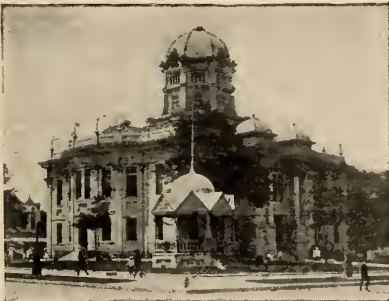
Marion County Court House.
