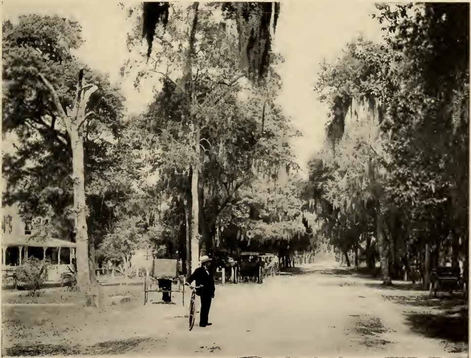
RIDGEWOOD AVENUE—DAYTONA. Copyright, 1904, by the Rotograph Co.
