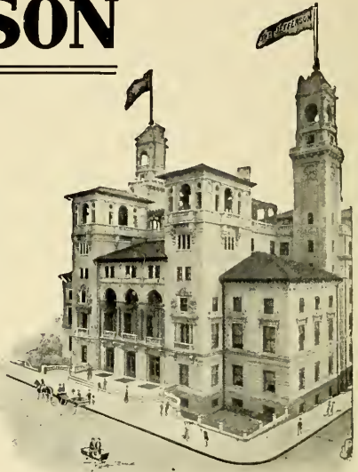
FRANKLIN STREET FRONT.
