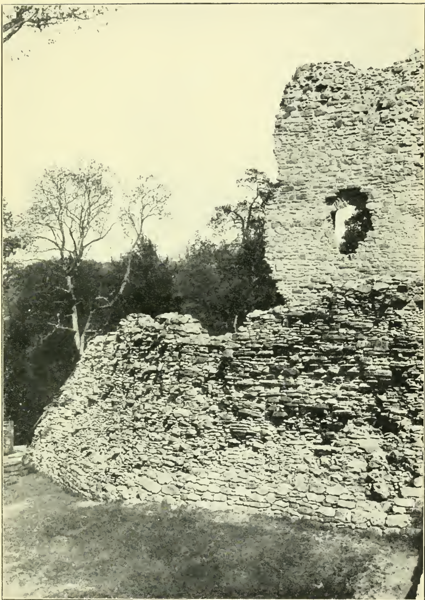
Fig. 15. The Welsh Tower, from the West Tower.
