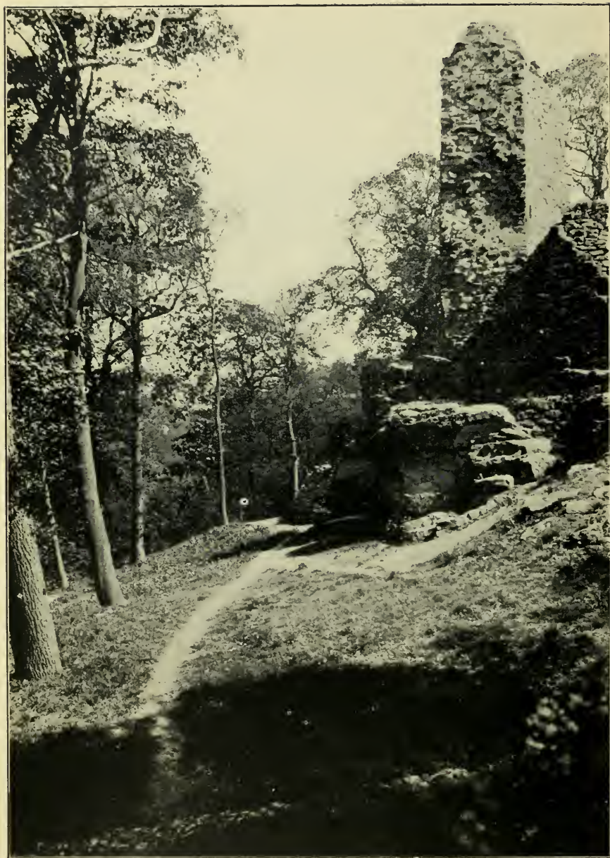
Fig. 18. The West Tower from the west.
