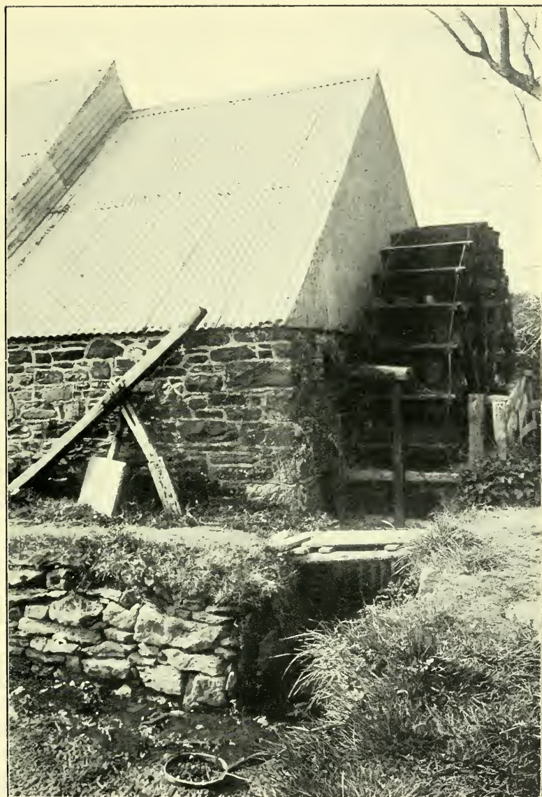
Fig. 5. The Llanrhystyd Yarn Factory. The undershot waterwheel and sluice-gate. Note the floodgate lever (which is manipulated from inside) projecting from the gable end of the building.
