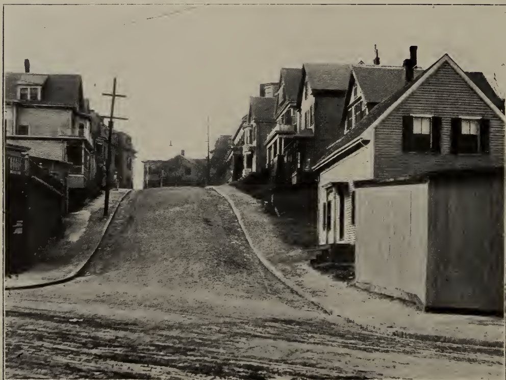
MYSTIC STREET AFTER ACCEPTANCE AND CONSTRUCTION.
