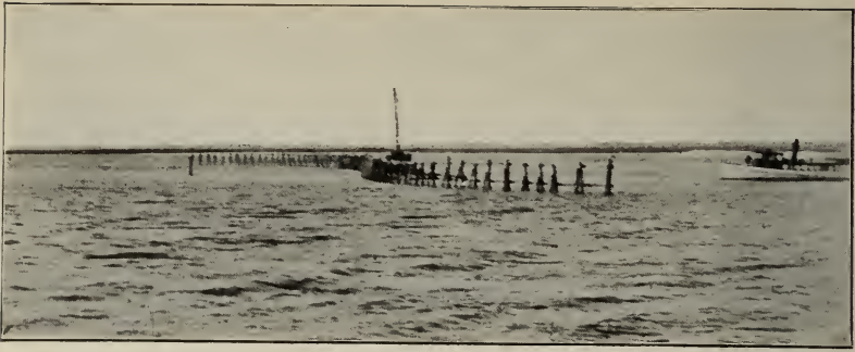
Fig. 1. Longport reaction jetty during construction.
