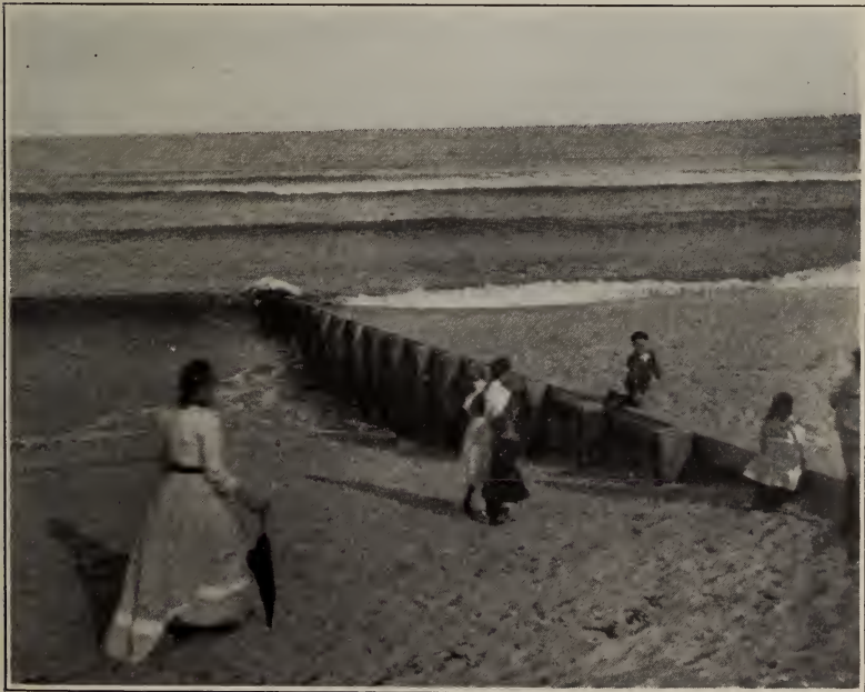
Fig. 2. A low groyne or jetty at Belmar.
