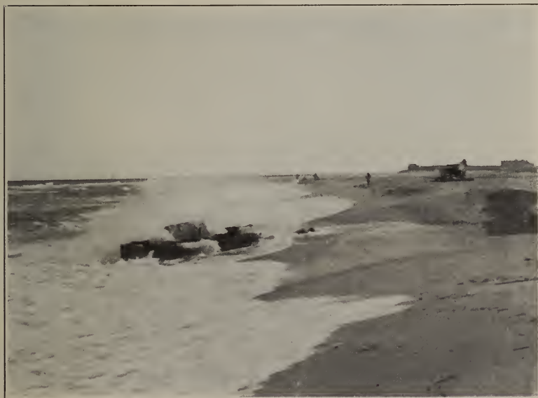
Fig. 2. Effect of a wreck at Squan River in causing erosion of the shore.
