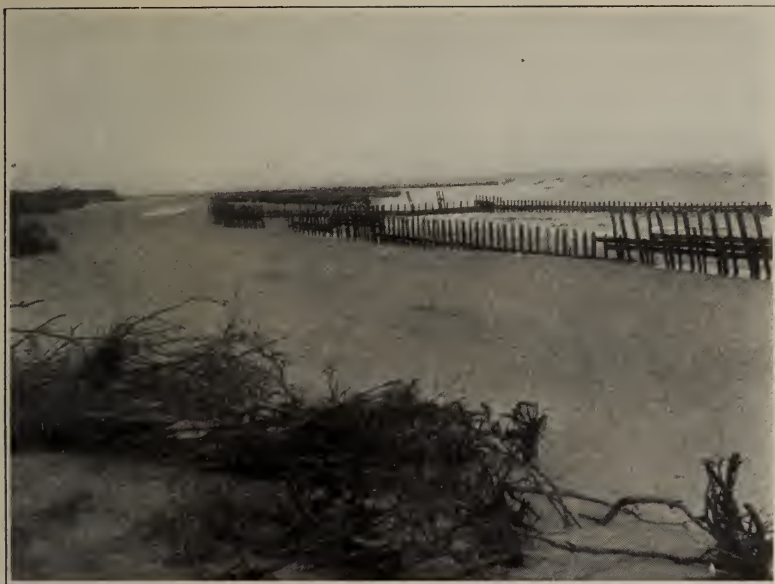
Fig. 1. Sand fences at Longport.
