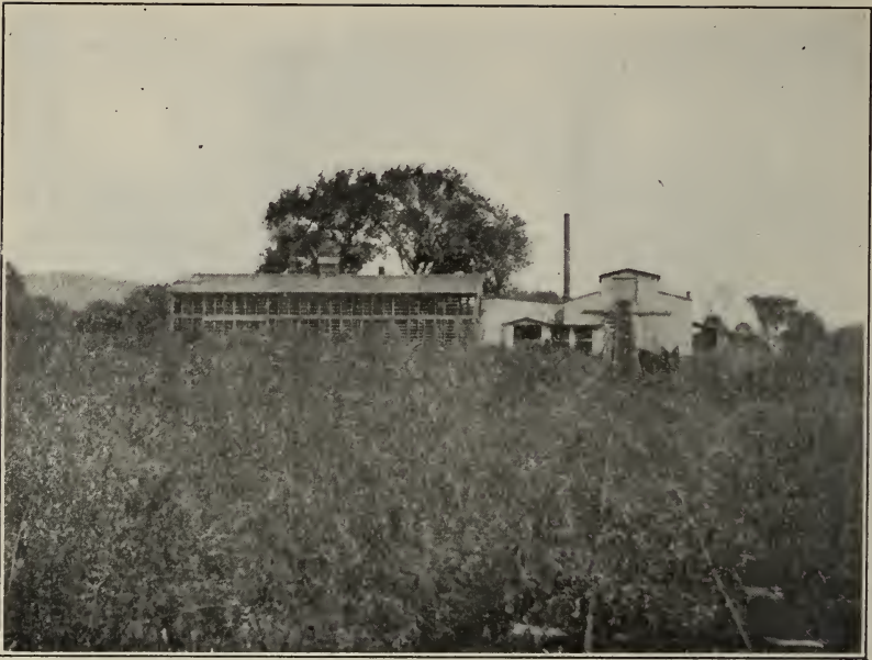
Fig. 1. General view of plant of American Peat Coal Company. The drying house, main building and track from the pits to the bins are shown.
