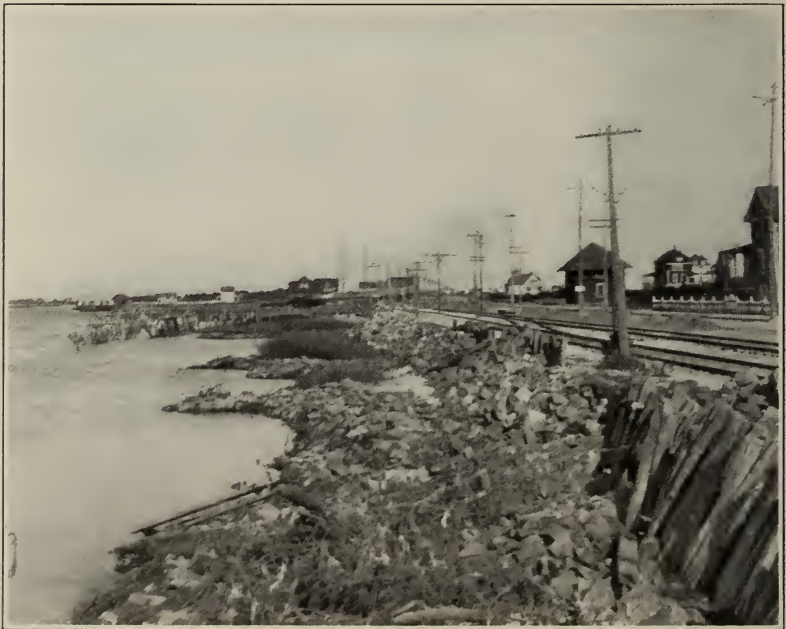
Fig. 2. The same after refilling and building stone revetment.
