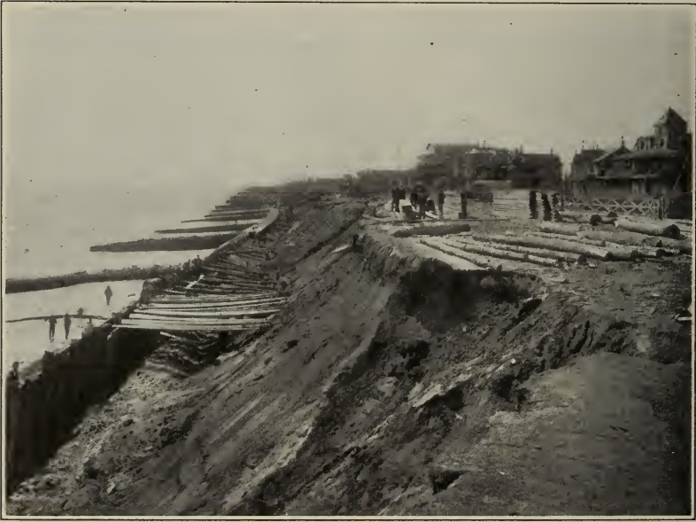
Jetties and bulkhead at Long Branch.
