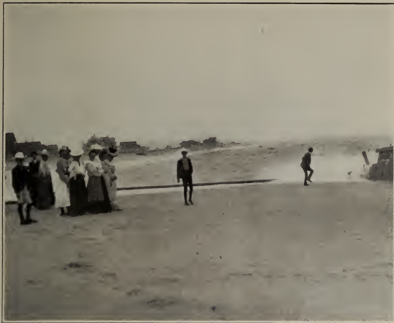
Fig. 1. Effect of a wreck at Sea Side Park in building out the shore.
