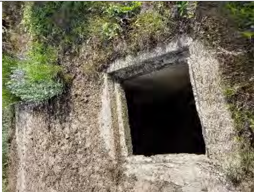
Photo 39. Looking into concrete basin.
