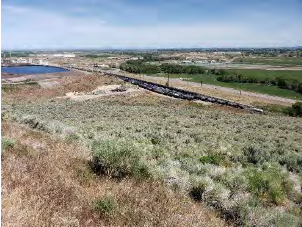
Photo 5. Looking northeast at railroad tracks (Don Plant on the left side of the photo).
