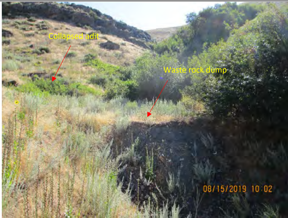
Photo 16. Additional abandoned mine features were observed, but not considered physical safety hazards. A collapsed adit and waste rock dump was also observed at: 42.809979°, -112.324790°. View of collapsed adit and waste rock dump looking east up drainage. Photograph taken by Bryce Anderson 8/15/2019.
