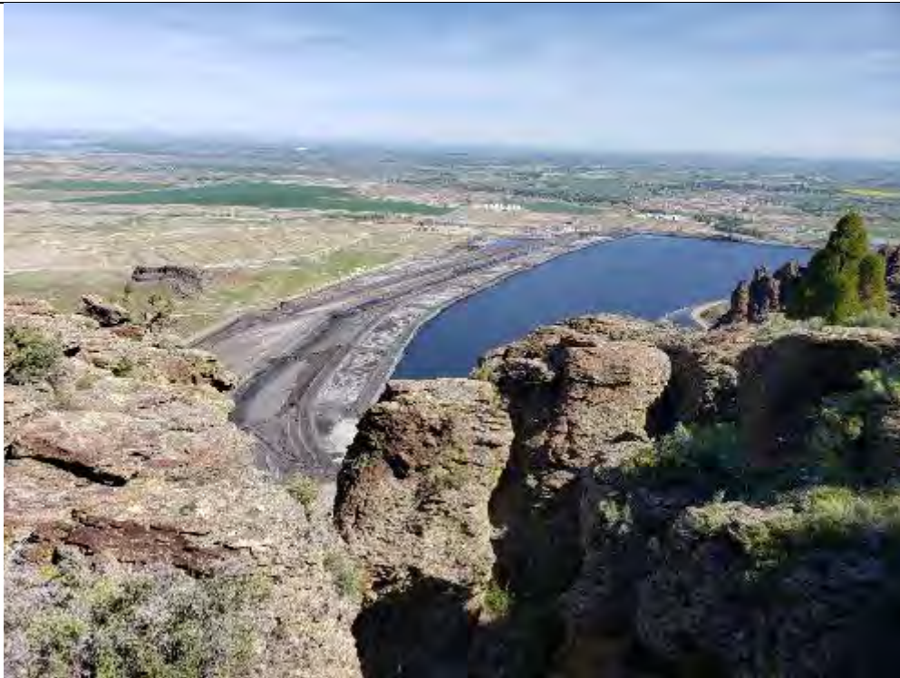
Photo 4. Looking north across Don Plant gypsum stack.
