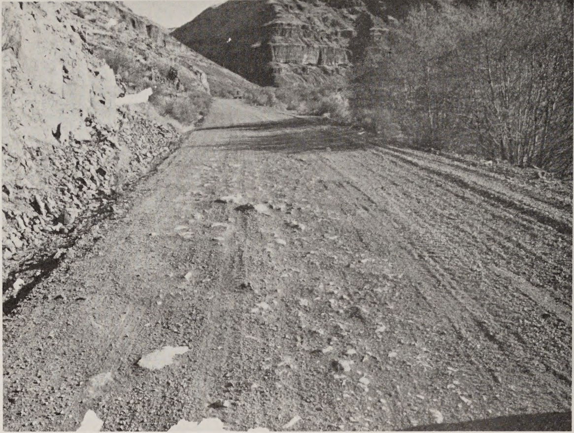
TYPICAL AREAS OF DETERIORATING ROAD SURFACE
