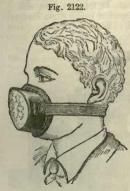
solution of caustic potash in a tube, as devised by Mitscherlich and modified by De Koninck. Air containing a dangerous proportion of carbonic oxide is fit for respiration after passing through the potash solution. A valve arrangement ensurcs inspiration of the cleansed air through the mouth, and expiration through the nose.
