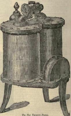
haust steam, producing a continuous suction and rise of water and a steady stream of water, two suction pumps may be combined, the steam entering alternately the one and then the other, while this admission may be regulated in the same way as represented in Fig. 2495, or by means of other power, when the pulley is driven by a belt from shafting above.
