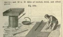
Imitation of Tile Pavement in Asphalt Coulé (Carrelages).
