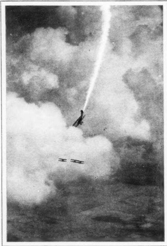
Trailing a Streamer of Smoke, a Cabinet Plane Dives Out of the Clouds to Start a Dog Fight with Three Enemy Ships
