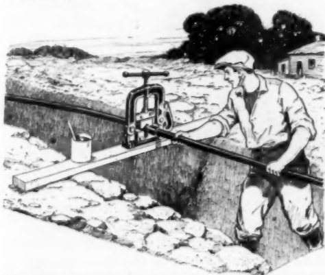
Pipe Vise Clamped on Plank Aids Worker to Lay Piping Single-Handed
