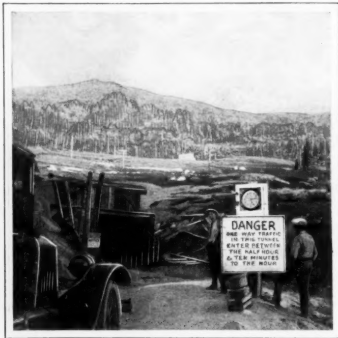
At Entrance to Old Railway Tunnel Now Used by Automobiles; the Clock and Sign Help Regulate One-Way Traffic
