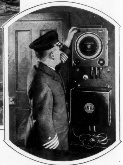
The Electric Sounder, Above, Has Replaced the Lead; at Right, the Indicator Which Shows the Sea Depth
