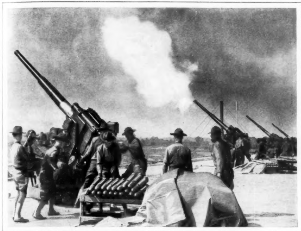
Anti-Aircraft Guns Which Aim Themselves, Being Tested at Aberdeen Proving Ground; a Sensitive Sound Pick-Up Points the Weapon Directly at the Source of the Sound
