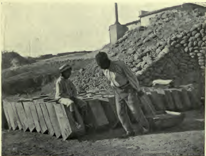
"WOODEN MOULD CONTAINING LIQUID SULPHUR." (Page 183.)
