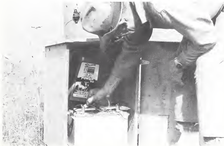
Skunk Creek Company Ranch Manager Bill Golladay connects energizer to 12-volt wet cell battery powering a 2-wire electric fence. Notice ground rod at left.
