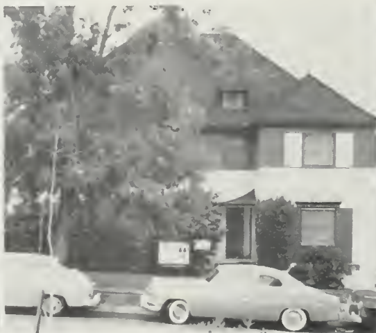
LANDFAIR HOUSE 500 Landfair Avenue
