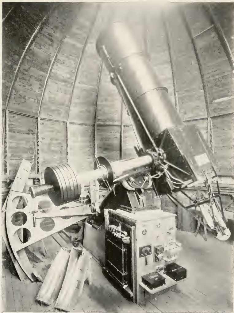
PLATE XXVI. THE 37-INCH MILLS REFLECTOR, SANTIAGO, CHILE.
