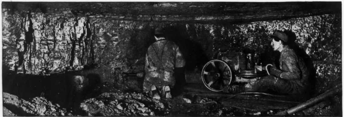
One of the fifteen Electric Punchers operated by the Berwind-White Coal Mining Co. at Windber, Pennsylvania.
