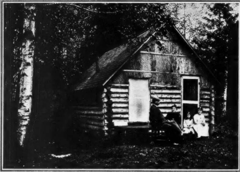
Vacation Log Cabln In Connecticut
