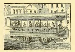
It is claimed that a car mile may be run on two gallons of liquid ammonia which iu turn requires four pounds of coal for its formatiou; and that ou a road rnnning fifty cars they may be operated for \$2.40 per day each.
